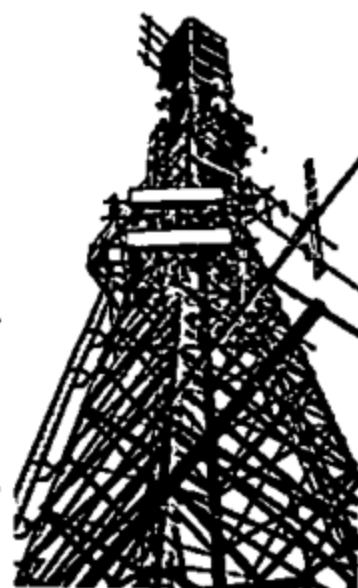
UHF receiving aerials (white rectangles) on a British local TV relay transmitter
